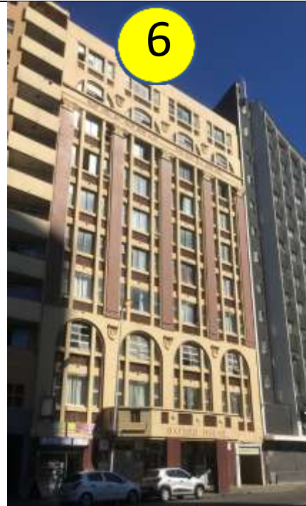
Oxford House 77 Gillespie Street (1933 in the Natal Mercury) Strange mixture of Classical Revival and Art Deco
