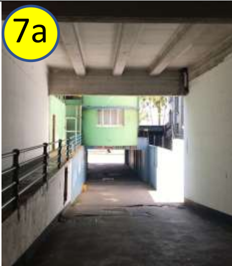
Driveway passing under Devonshire Court
