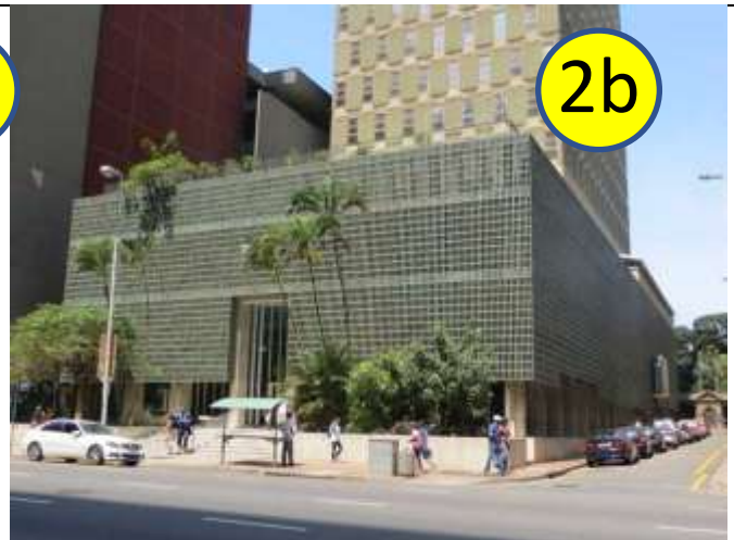
The Nedbank building is distinguished by the travertine podium to the pavement, water fountains and vegetation, its diminutive scale, the suspended filigree screen shielding the interior from the inclement effects of the sun, and a roof garden (which is currently deserted)
