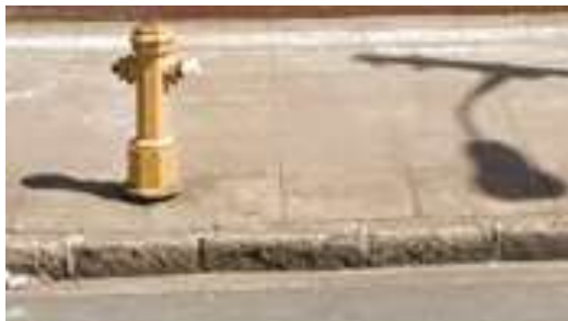
Old stone kerbs for sidewalk outside Glenariff, 96 Umbilo Road
